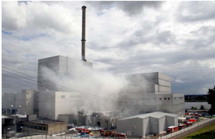
Figure 11. Fire extinguishing activities supported by the external local fire fighters
