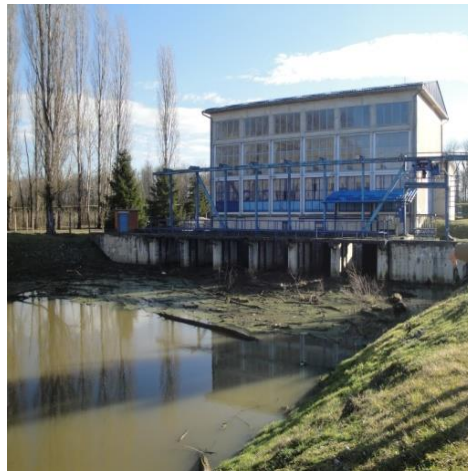
Figure 3: Drainage water collected from wider ameliorated area in the main canal and pump's wet well
