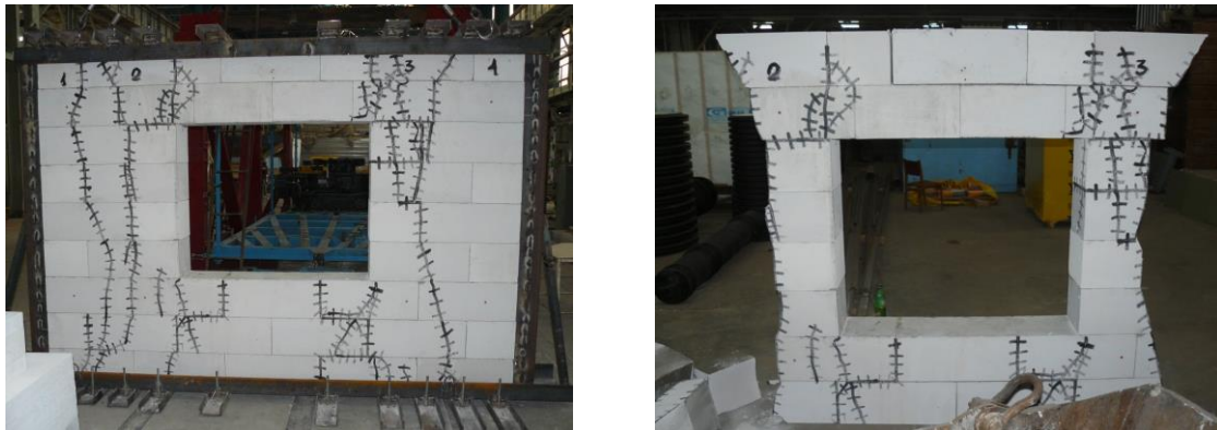
Fig. 11: The nature of the destruction of a non-reinforced panel made of cellular concrete blocks during dynamic tests
