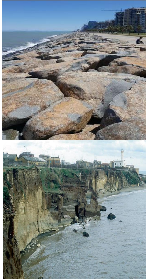
Figure 5: Covering massive boulders, protecting against the abrasive effects of waves (A); Result of the abrasive collapse of sea waves (B)
