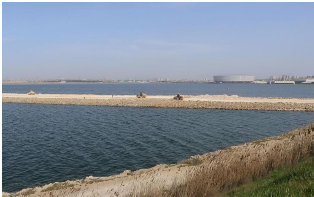
Figure 2: Photo of the dam construction process on Lake Boyuk-Shor
