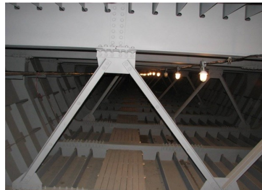
Picture 4: Internal structures of the bridge
