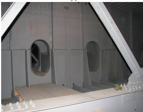
Picture 5: Transition bays between bridge sections at the piers
