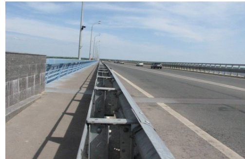
Picture 2: View of the roadway and pedestrian part of the bridge
