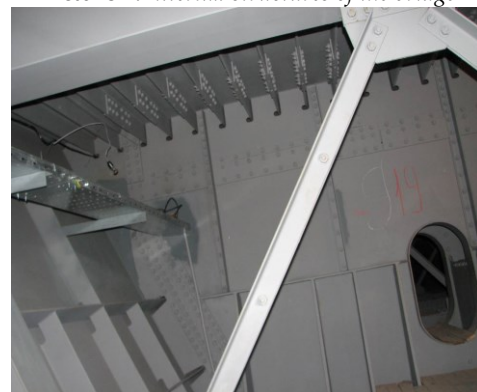
Picture 6: Internal construction of bridge span adjacency to piers
