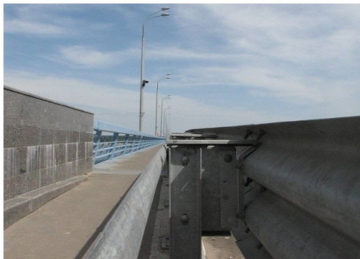
Picture 3: Roadway fence construction
