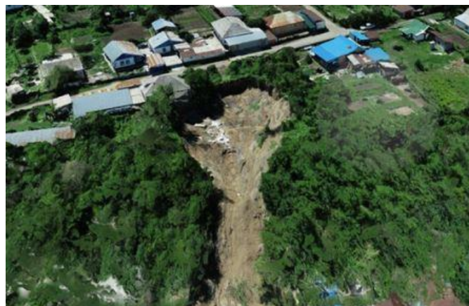
Fig. 1: General view of the landslide on 15.05.2022 in Tekeli
