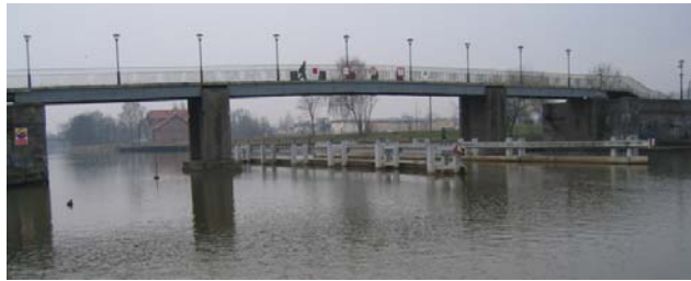
Figure 14. Lower bridge in Elblag
