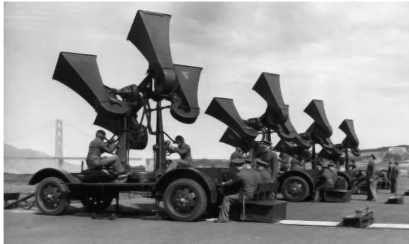
Figure 1: Acoustic detection complex based on ZT-5
